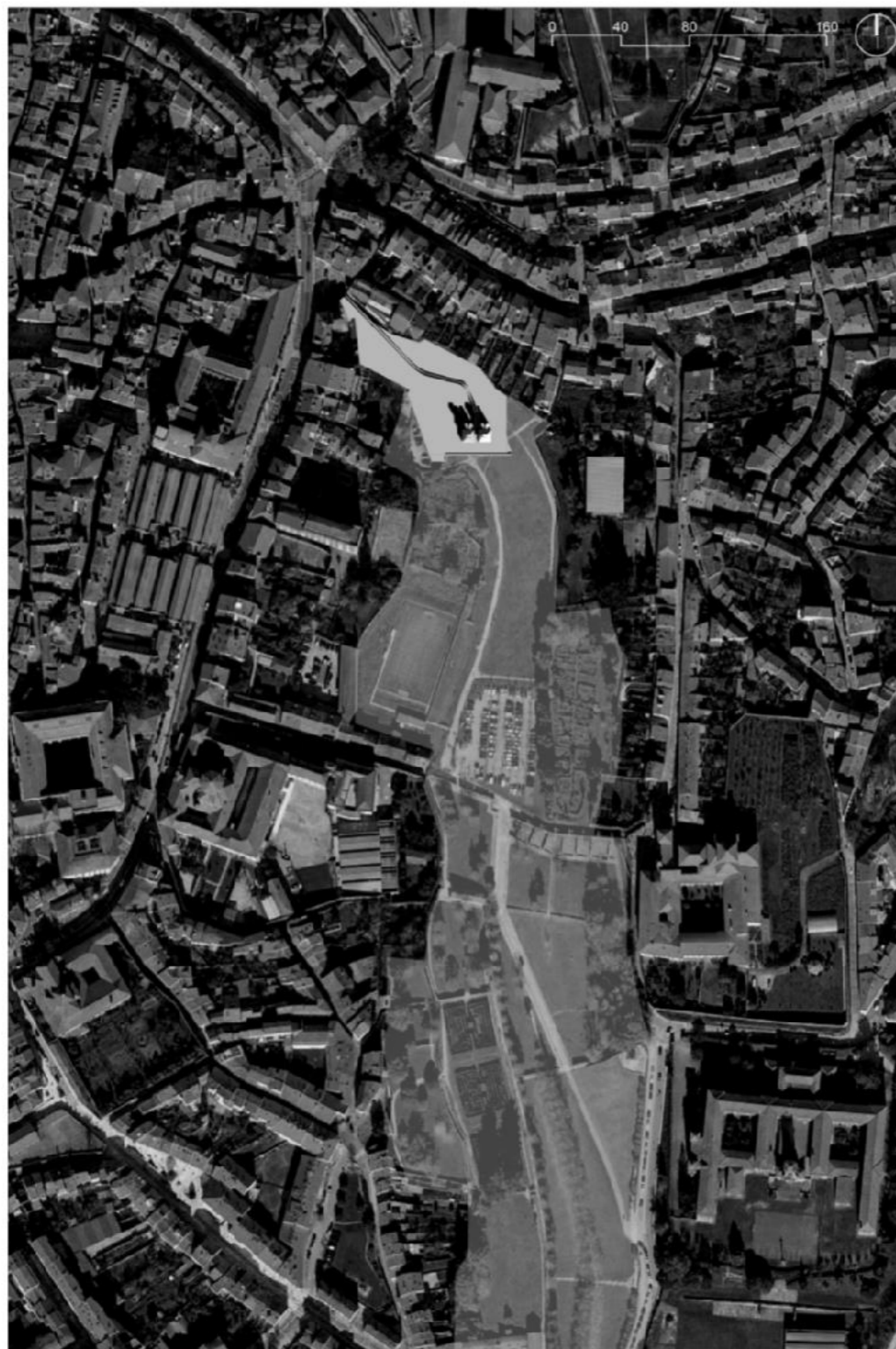
OVERVIEW Botanical Towers project settled in its original position on actual orthophoto.
